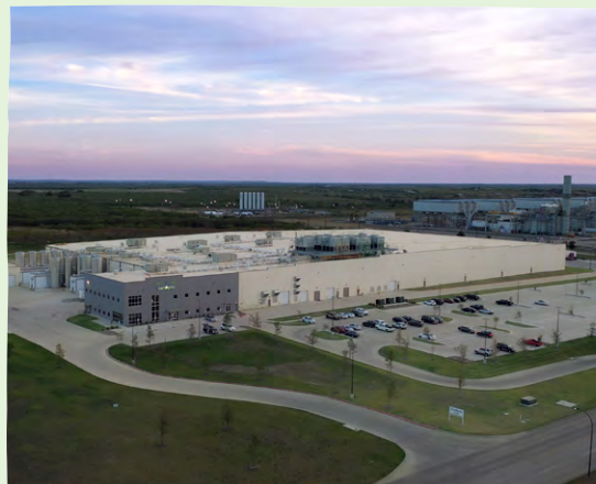
Our Texas plant was built with sustainability in mind.
